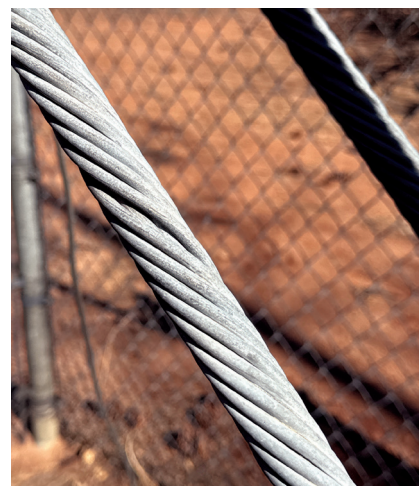
Fig. 5 — Closer view of one of the anchor CC guy wires clearly shows no exposure to wildfire.
