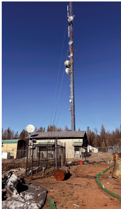
Fig. 1 — Telecommunications tower featured in this case study.
