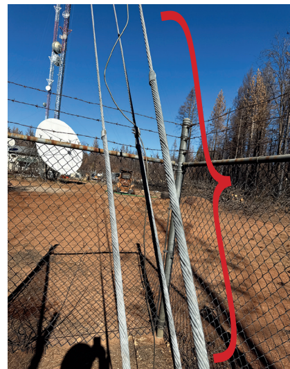
Fig. 3 — Photograph showing guy wires of anchor CC.
