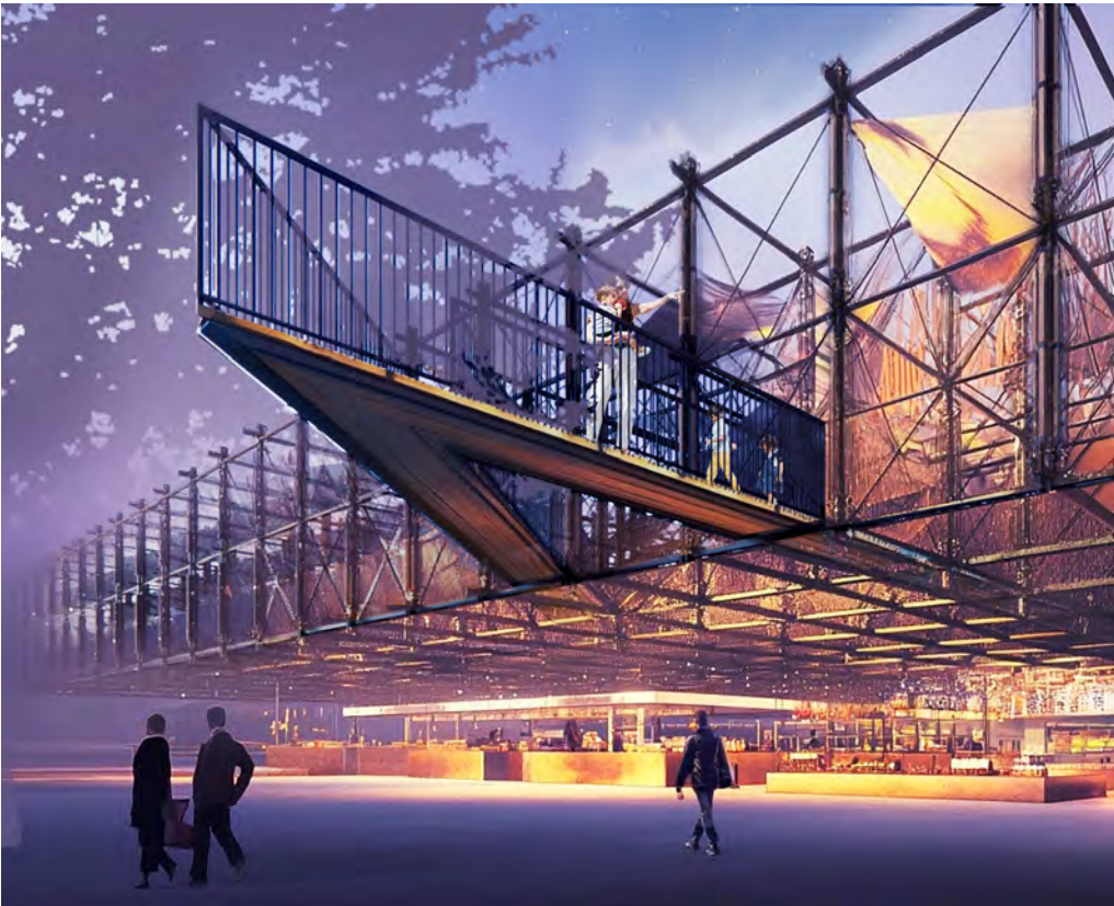
The final design by UT Austin architecture students Alexandr Terekhov and Andrew Blanco envisions a farmers market composed of modular tensegrity components that form a striking, large-scale shading structure.
