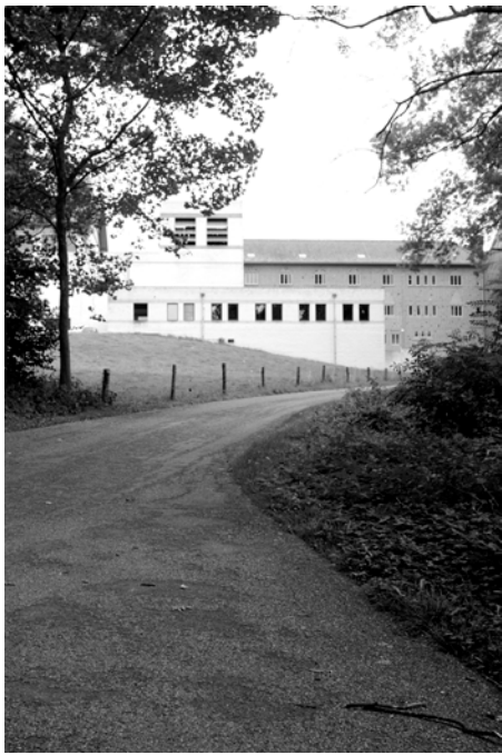
FIGURE 4. Exterior view of the St. Benedictusberg Abbey (1967-1986) at Mamelis (near Vaals), Netherlands, designed by Hans van der Laan.
