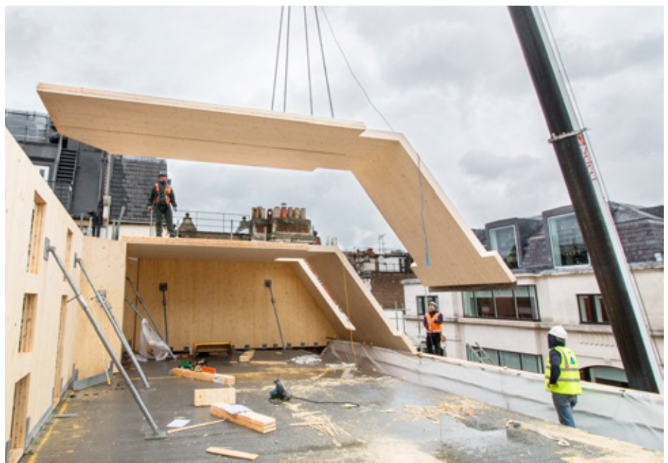
CLT used in a rooftop story extension. PHOTO: Courtesy of Eurban
