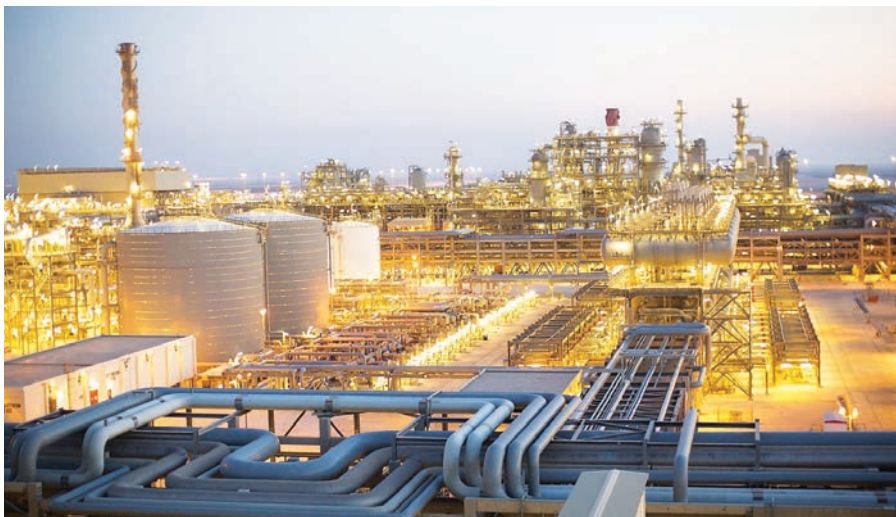
FIG. 1. View of the Pearl GTL plant. Photo courtesy of Shell.
