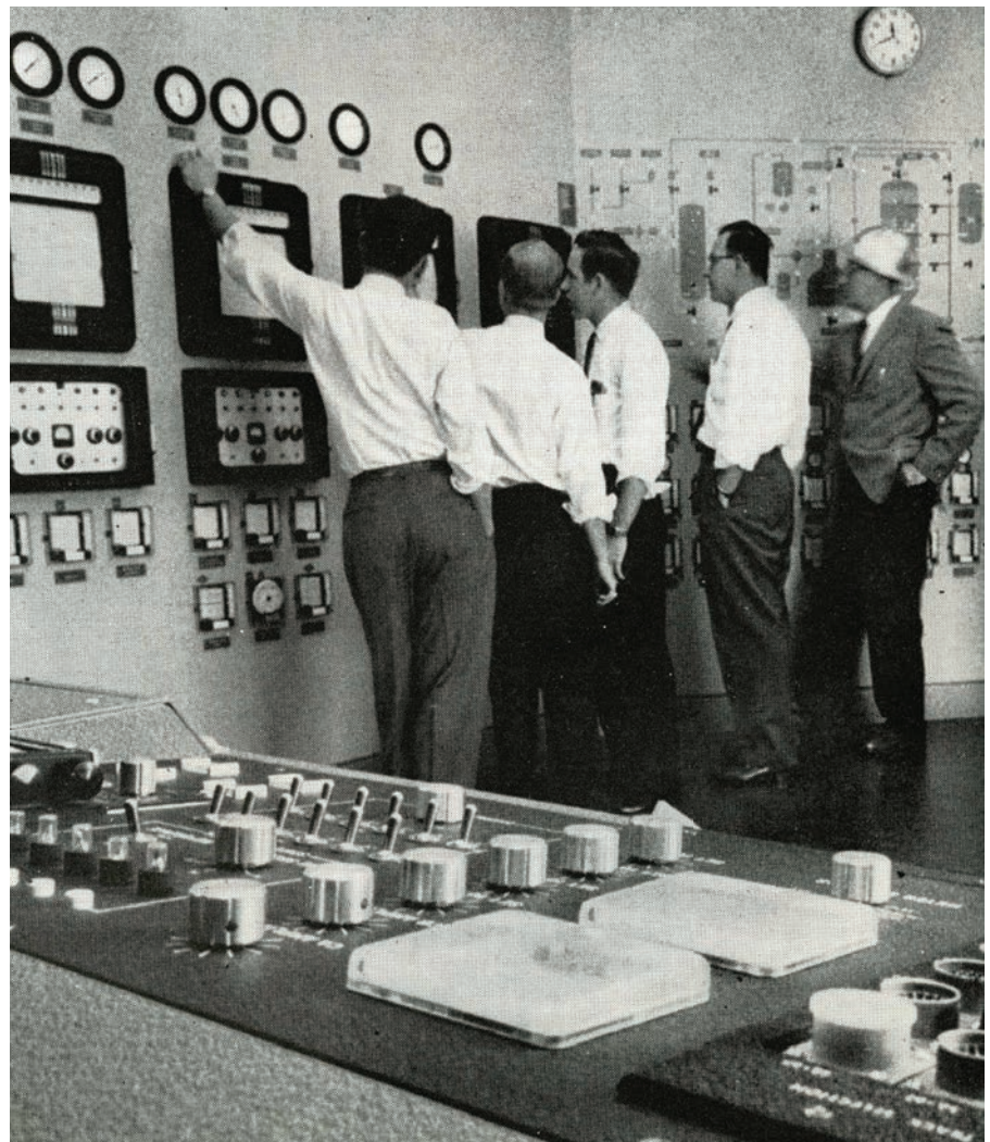
FIG. 4. The RW-300 computer system, foreground, was used to enhance operations at Texaco's Port Arthur refinery's 1,600-bpd polymerization plant. In the background, Texaco engineers and TRW personnel check control charts. Photo courtesy of Business Week .
