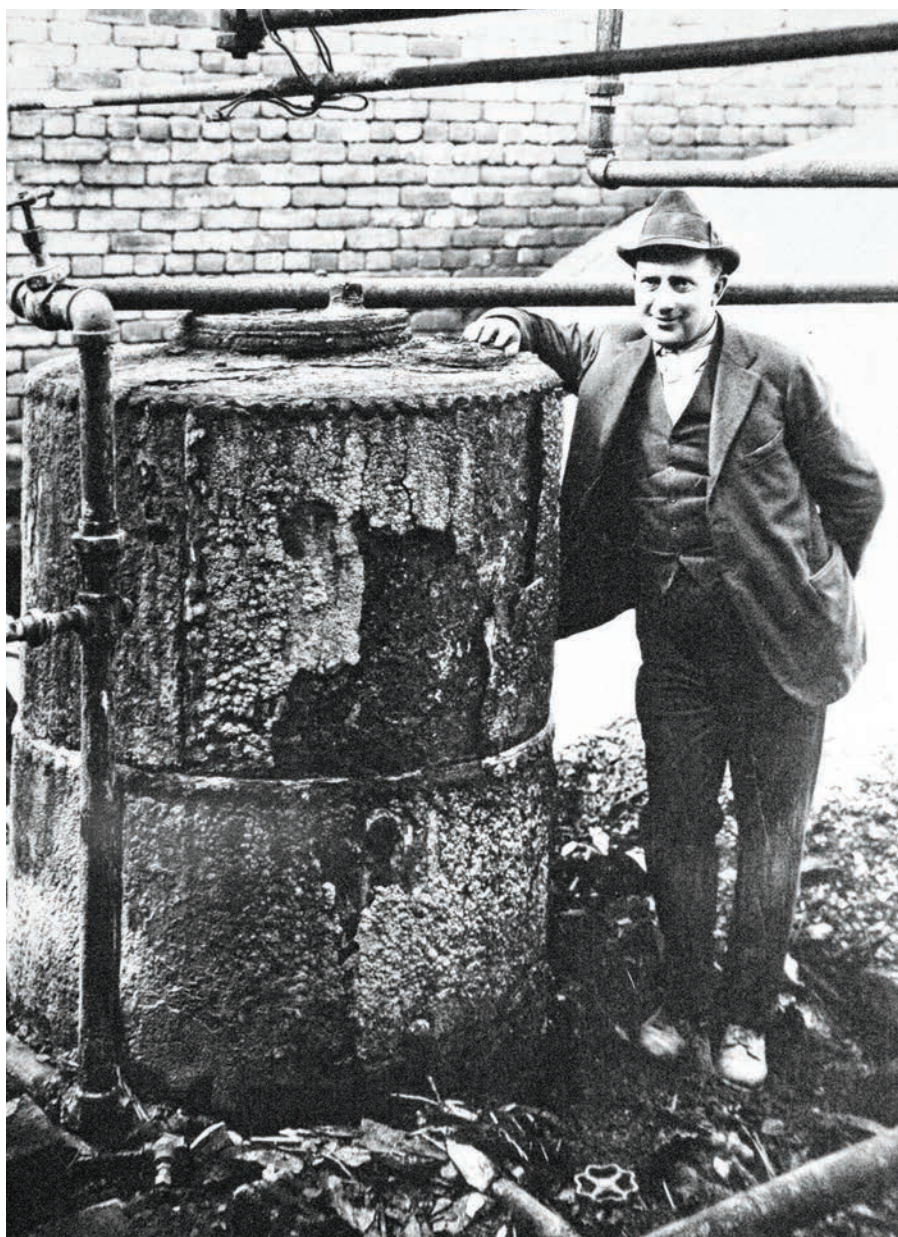
FIG. 1. Samuel Kier standing next to his 5-bpd petroleum still. Photo courtesy of the Drake Well Museum.
