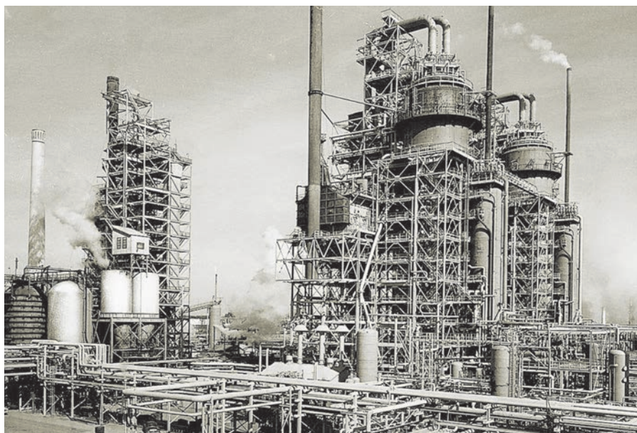
FIG. 1. View of Standard Oil of New Jersey's PCLA Model 1 plant in Baton Rouge, Louisiana—the first use of a commercial catalytic cracking process using powdered catalyst. Photo courtesy of the American Chemical Society.
