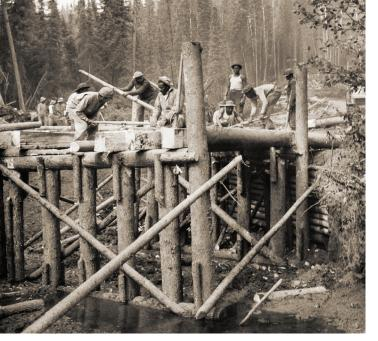
route. Many of these temporary bridges couldn't withstand the thawing of rivers in the spring, according to Rogers. "Flotsam in the form of tree trunks and brush ... slammed into the pilings, damaging them and capturing more and more debris because of the obstructions," he says.
