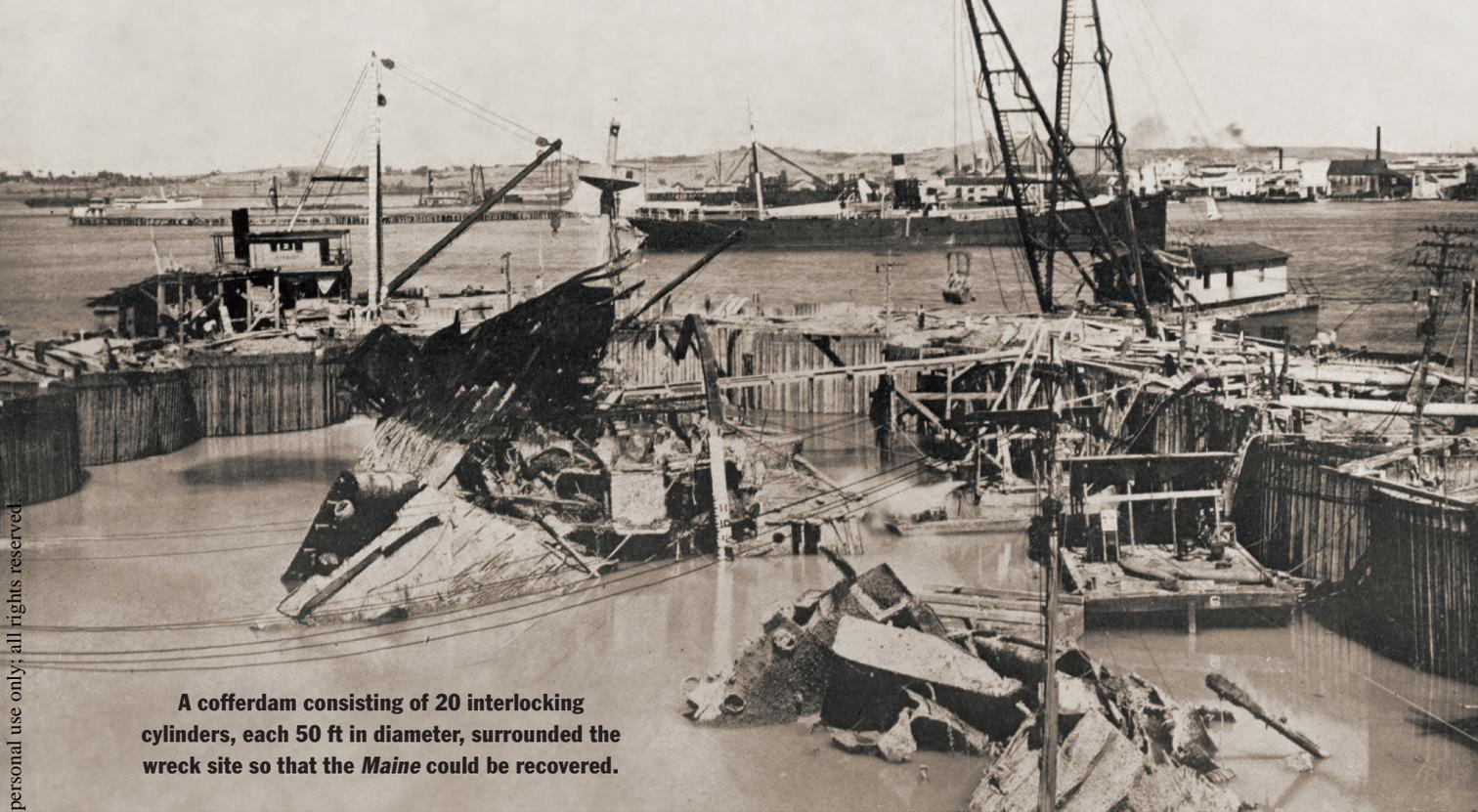
**A cofferdam consisting of 20 interlocking cylinders, each 50 ft in diameter, surrounded the wreck site so that the *Maine* could be recovered.**
