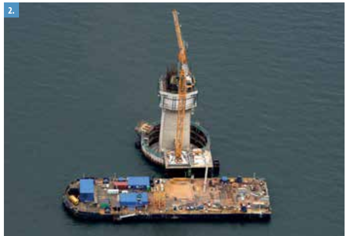
Images courtesy of Transport Scotland: 1. Construction of the towers has been achieved successfully despite occasional high winds for which the area is notorious 2. Concrete for the towers has been pumped from barges moored alongside 3. When the steelwork was pushed out towards the piers, the ends had to be raised to slide over the top 4. The bridge project is on track for completion at the end of 2016
