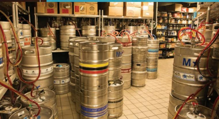
**World of Beer**, Tampa, Fla., stores kegs in a long, narrow cooler, tapping 50 brews through the wall to the bar. Another 12 travel through trunk lines to an upstairs bar serving an outdoor patio. The system is from Micro Matic.
