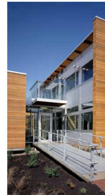
EXTERIOR SUNSHADES SEPARATE VISION GLAZING FROM DAYLIGHT GLAZING TO ASSIST IN DAYLIGHT HARVESTING AND GLARE CONTROL. [IMAGE COURTESY OF BP+W]
