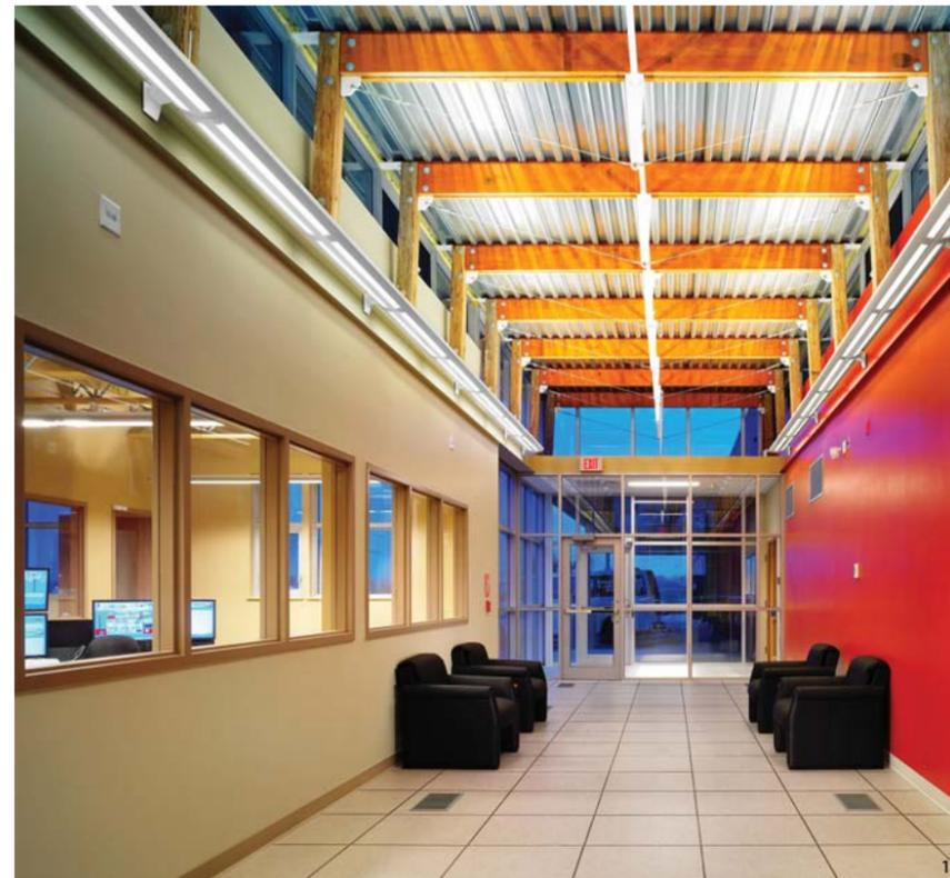
THE STRUCTURAL STEEL FRAME USES ALL BOLTED CONNECTIONS. OPEN WEB STEEL JOISTS HAVE A WOOD TOP CHORD TO PERMIT SCREW FASTENING OF THE METAL DECK. LATERAL RESISTANCE IS PROVIDED BY HEAVY GAUGE STEEL STUDS MECHANICALLY FASTENED TOP AND BOTTOM. MASONRY VENEER AND STUCCO PANELS ARE MECHANICALLY FASTENED BACK TO THE STRUCTURE. WOOD SIDING IS FASTENED WITH SCREWS. DESIGN: MCCALLUM SATHER ARCHITECTS, HAMILTON, ON
