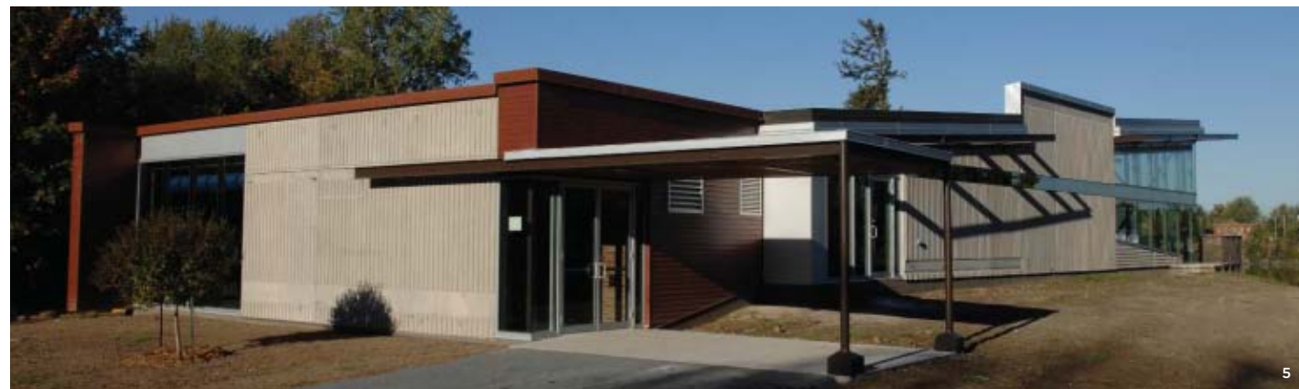
FOR THE POINTE VALAINE COMMUNITY CENTRE IN OTTERBURN PARK QC, ARCHITECTS SMITH VIGEANT USED 13 PRECAST CONCRETE INSULATED PANELS SALVAGED FROM THE RETROFIT OF TWO NEARBY CANADIAN TIRE STORES. TOTALING ABOUT 35M 2 OF CONCRETE, THE PANELS MAKE UP MORE THAN 40% OF THE EXTERIOR WALLS. THE PANELS WERE TRIMMED TO THE REQUIRED LENGTH BY GROUPE TREMCA , BUT RETAIN THE ORIGINAL CONNECTION DETAIL AT THE TOP. FOR MORE ON THIS PROJECT SEE SABMAG ISSUE 18.
