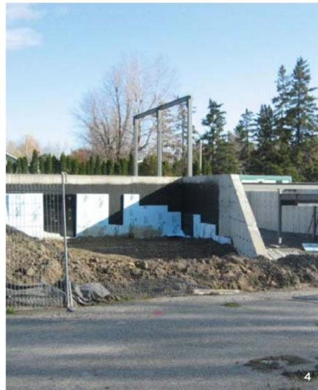
FOR THE POINTE VALAINE COMMUNITY CENTRE IN OTTERBURN PARK QC, ARCHITECTS SMITH VIGEANT USED 13 PRECAST CONCRETE INSULATED PANELS SALVAGED FROM THE RETROFIT OF TWO NEARBY CANADIAN TIRE STORES. TOTALING ABOUT 35M<sup>2</sup> OF CONCRETE, THE PANELS MAKE UP MORE THAN 40% OF THE EXTERIOR WALLS. THE PANELS WERE TRIMMED TO THE REQUIRED LENGTH BY GROUPE TREMCA , BUT RETAIN THE ORIGINAL CONNECTION DETAIL AT THE TOP. FOR MORE ON THIS PROJECT SEE SABMAG ISSUE 18.
