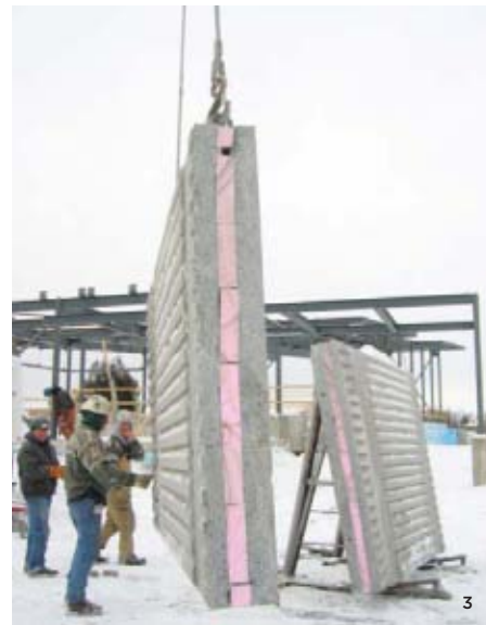
FOR THE POINTE VALAINE COMMUNITY CENTRE IN OTTERBURN PARK QC, ARCHITECTS SMITH VIGEANT USED 13 PRECAST CONCRETE INSULATED PANELS SALVAGED FROM THE RETROFIT OF TWO NEARBY CANADIAN TIRE STORES. TOTALING ABOUT 35M 2 OF CONCRETE, THE PANELS MAKE UP MORE THAN 40% OF THE EXTERIOR WALLS. THE PANELS WERE TRIMMED TO THE REQUIRED LENGTH BY GROUPE TREMCA , BUT RETAIN THE ORIGINAL CONNECTION DETAIL AT THE TOP. FOR MORE ON THIS PROJECT SEE SABMAG ISSUE 18.
