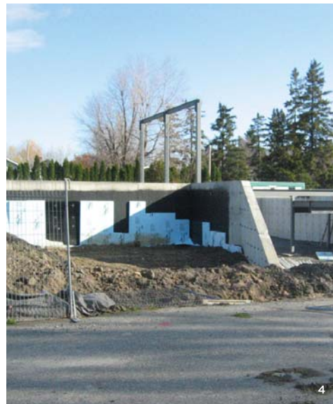
FOR THE POINTE VALAINE COMMUNITY CENTRE IN OTTERBURN PARK QC, ARCHITECTS SMITH VIGEANT USED 13 PRECAST CONCRETE INSULATED PANELS SALVAGED FROM THE RETROFIT OF TWO NEARBY CANADIAN TIRE STORES. TOTALING ABOUT 35M 2 OF CONCRETE, THE PANELS MAKE UP MORE THAN 40% OF THE EXTERIOR WALLS. THE PANELS WERE TRIMMED TO THE REQUIRED LENGTH BY GROUPE TREMCA , BUT RETAIN THE ORIGINAL CONNECTION DETAIL AT THE TOP. FOR MORE ON THIS PROJECT SEE SABMAG ISSUE 18.
