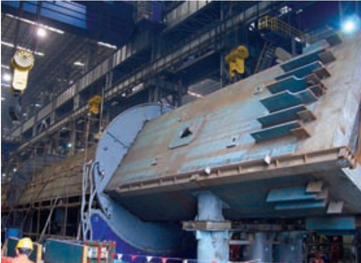
Tower unit being fabricated on the rotating jig.
