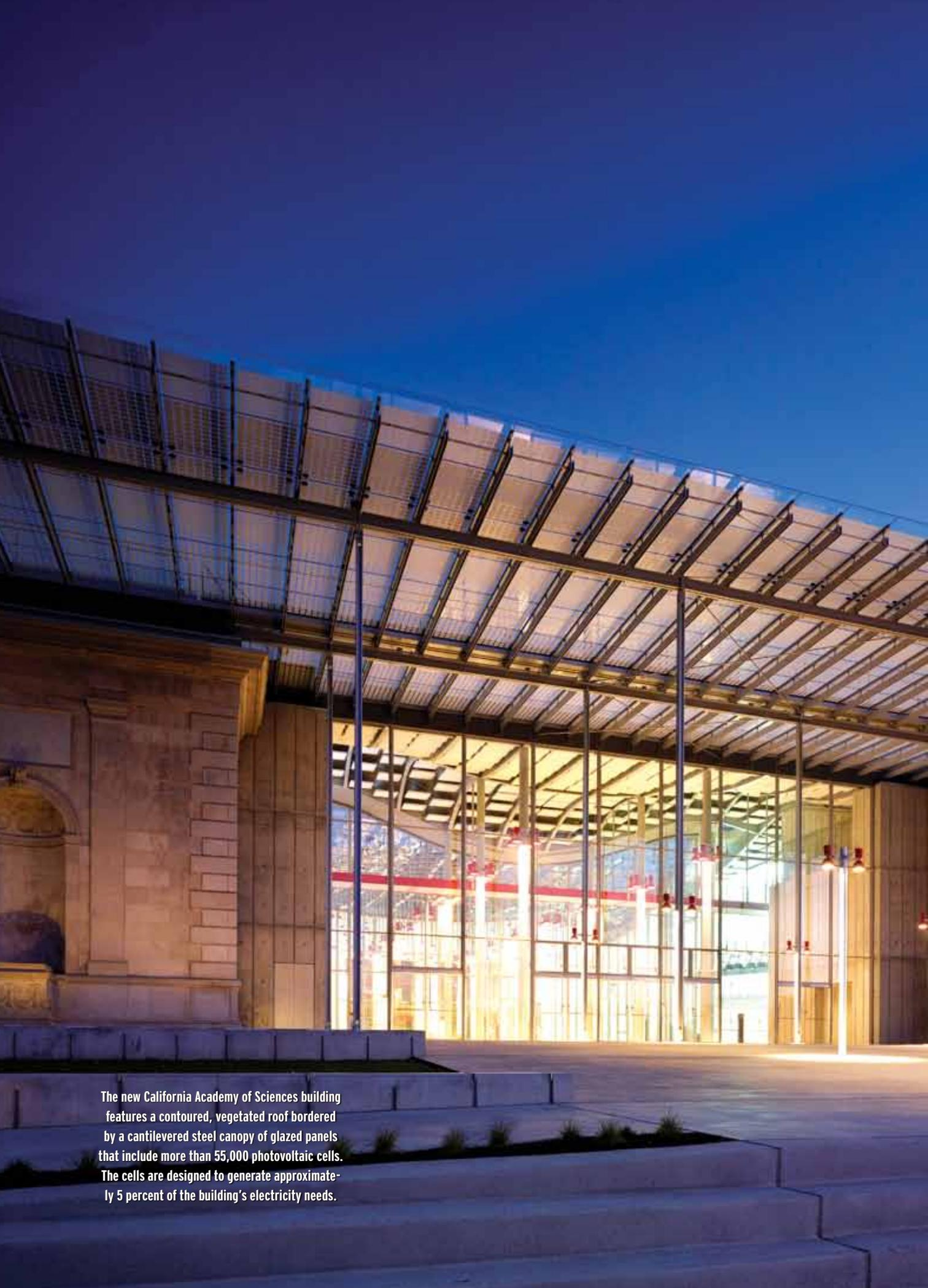
The new California Academy of Sciences building features a contoured, vegetated roof bordered by a cantilevered steel canopy of glazed panels that include more than 55,000 photovoltaic cells. The cells are designed to generate approximately 5 percent of the building's electricity needs.
