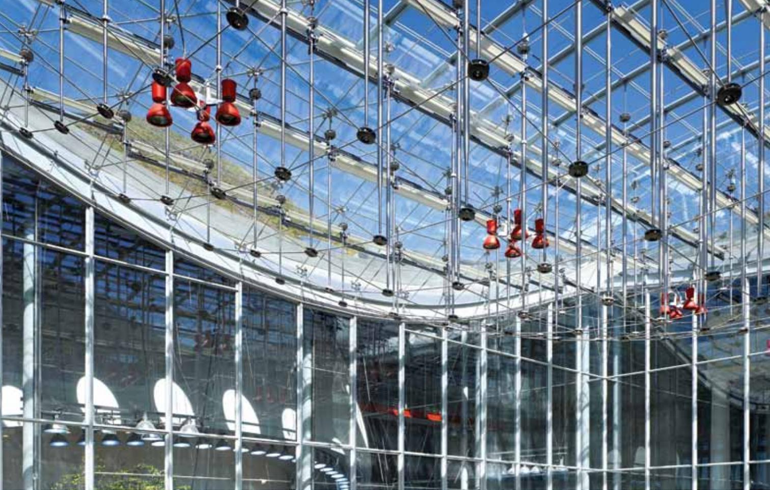
12 ft (3.7 m) in the center of that three-story space. Each round, articulated node consists of six elements—a housing, a spherical bearing for each of the four intersecting rods, and a machined ball into which the vertical strut is threaded—that were designed to “follow all the various changing geometries” of the twin nets, says Chambers.
